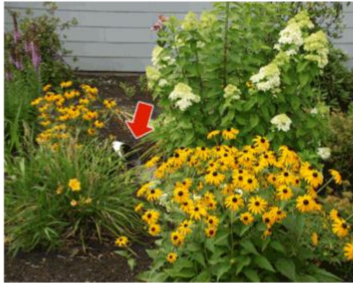
Downspout disconnection heading to the creek. Photo by Environmental Protection Agency. Public Domain. Available at: http://www.ellerbecreek.org/en/act/be-creek-smart/103-act/creek-smart/174-disconnect-your-roof-from-the-creek.html
